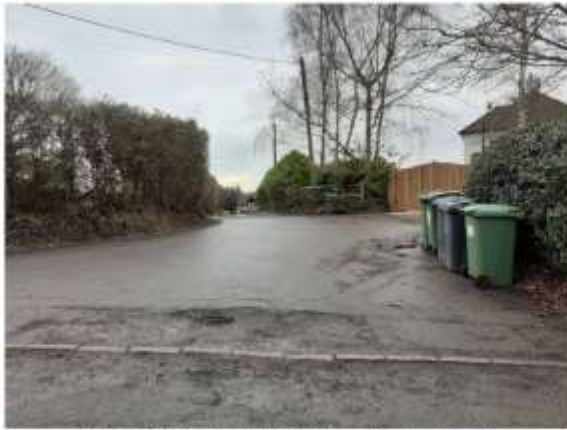
2023,7th March, Cold5-26 junction looking N
