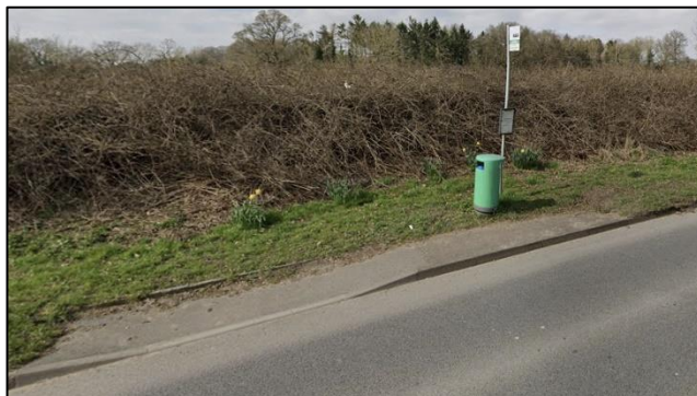
Bus stop at Cold Ash Hill with no shelter or pavement
